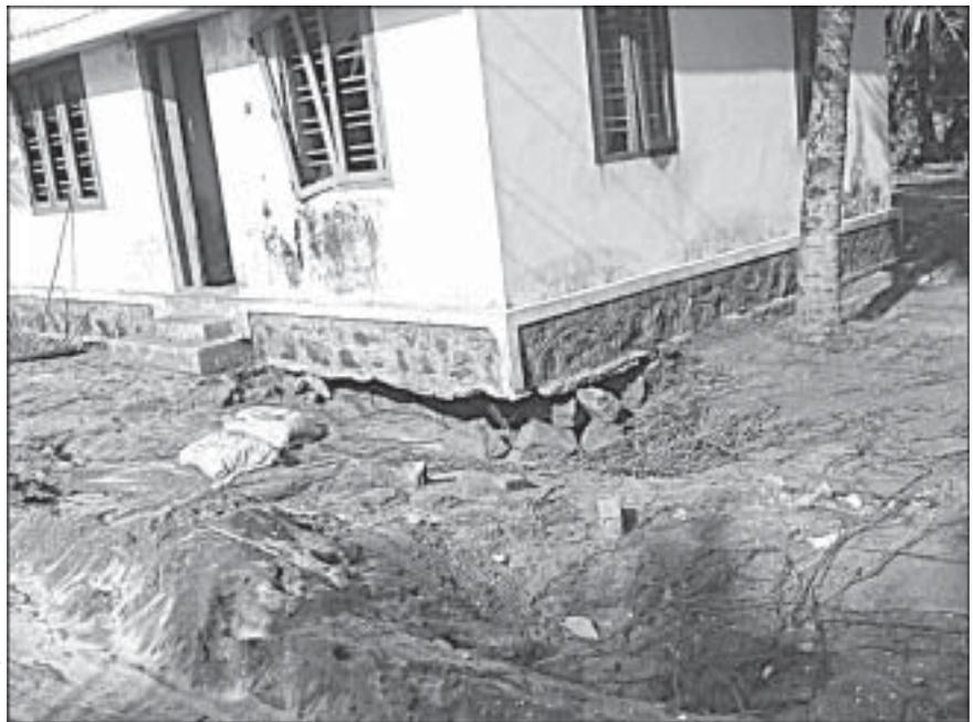
**Fig 9 Foundation failure in Kerala due to scouring of rather shallow foundation** (Photo: Alpa Sheth )
