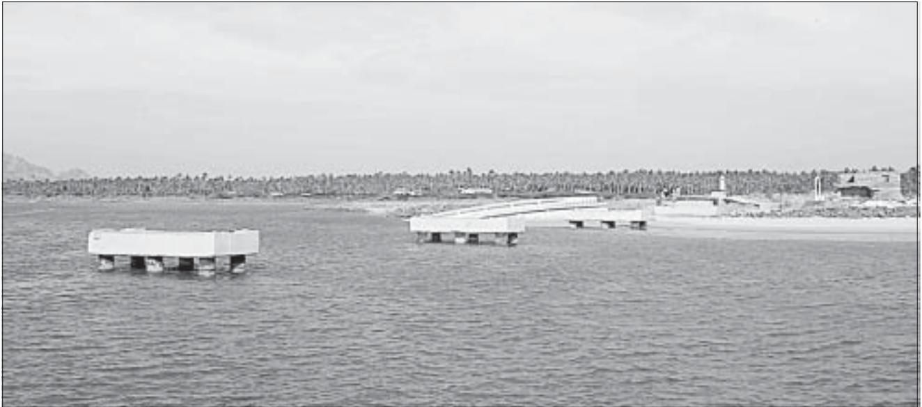
**Fig 10 Complete loss of the four span of a RC bridge at Melmannakudi** (Photo: Alpa Sheth)
