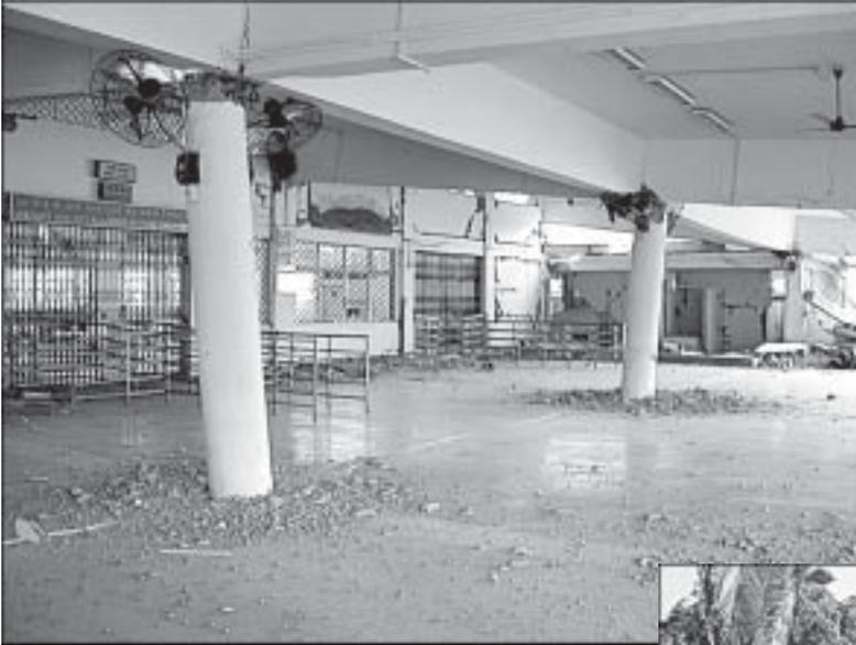
**Fig 2 Severe damage to Passenger Terminal Building at Port Blair** (Photo: Sudhir K Jain)
