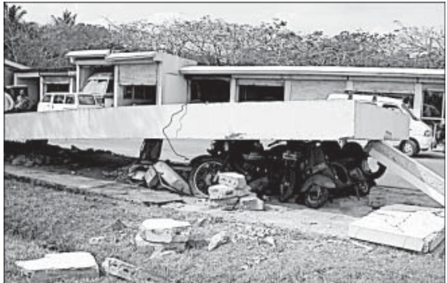
**Fig 5 Collapse of a reinforced concrete scooter stand at Port Management Board office in Port Blair** (Photo: Hemant Kaushik)
