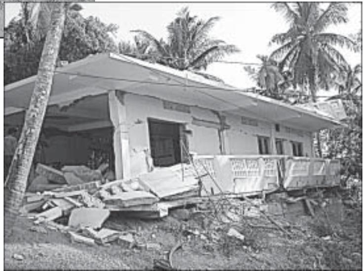
**Fig 4 Collapse of a stilt plus one-storey house in reinforced concrete near Port Blair** (Photo: Hemant Kaushik)
