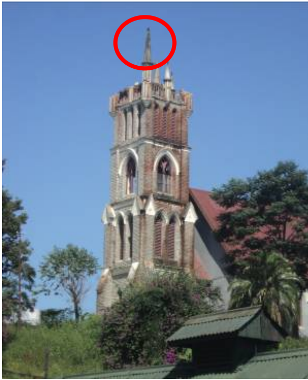
Fig. 19. Collapse of brick spires of Mac Farlene Church at Kalimpong (Photo: Keya Mitra)
