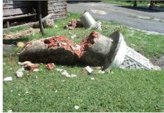
Fig. 19. Collapse of brick spires of Mac Farlene Church at Kalimpong (Photo: Keya Mitra)
