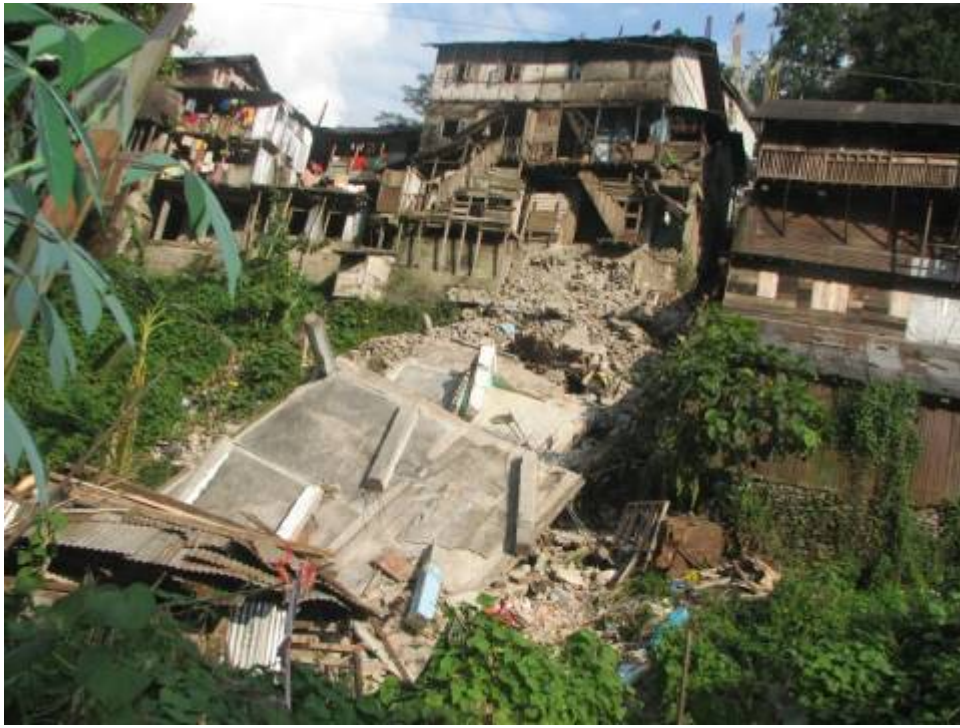
Fig. 8. Collapsed four story reinforced concrete building at Dikchu Bazaar (Photo: Hemant Kaushik)
