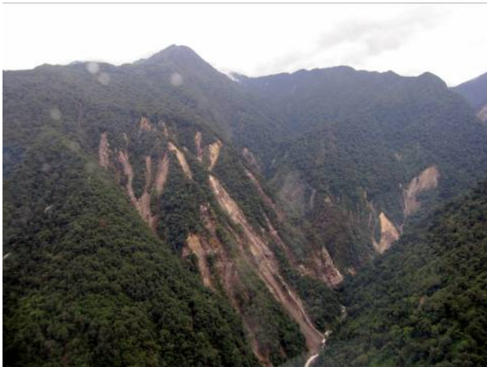
Fig. 5. Aerial photograph showing typical landslides enroute from Mangan to Chungthang and Lachung (Photo: Durgesh Rai)
