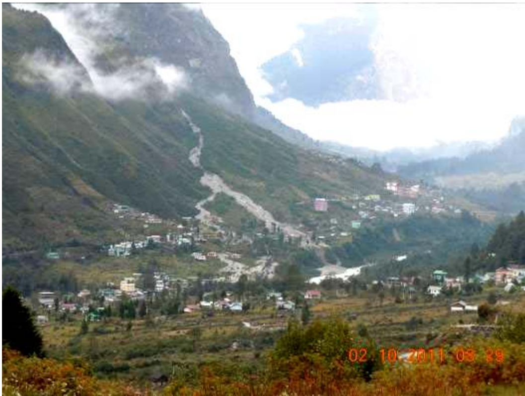
Fig. 4. Photograph of town Lachung showing massive rockslides (Photo: Vaibhav Singhal)
