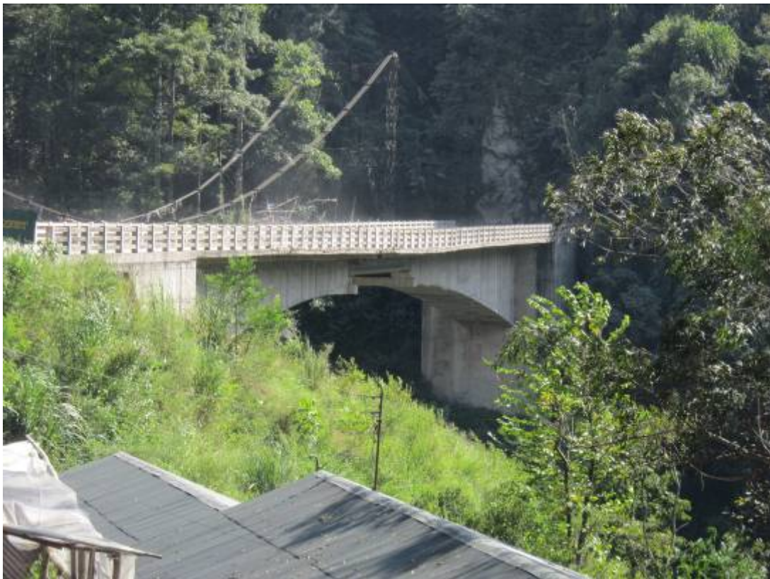
Fig. 16. Undamaged concrete bridge in North Sikkim (Photo: Durgesh Rai)
