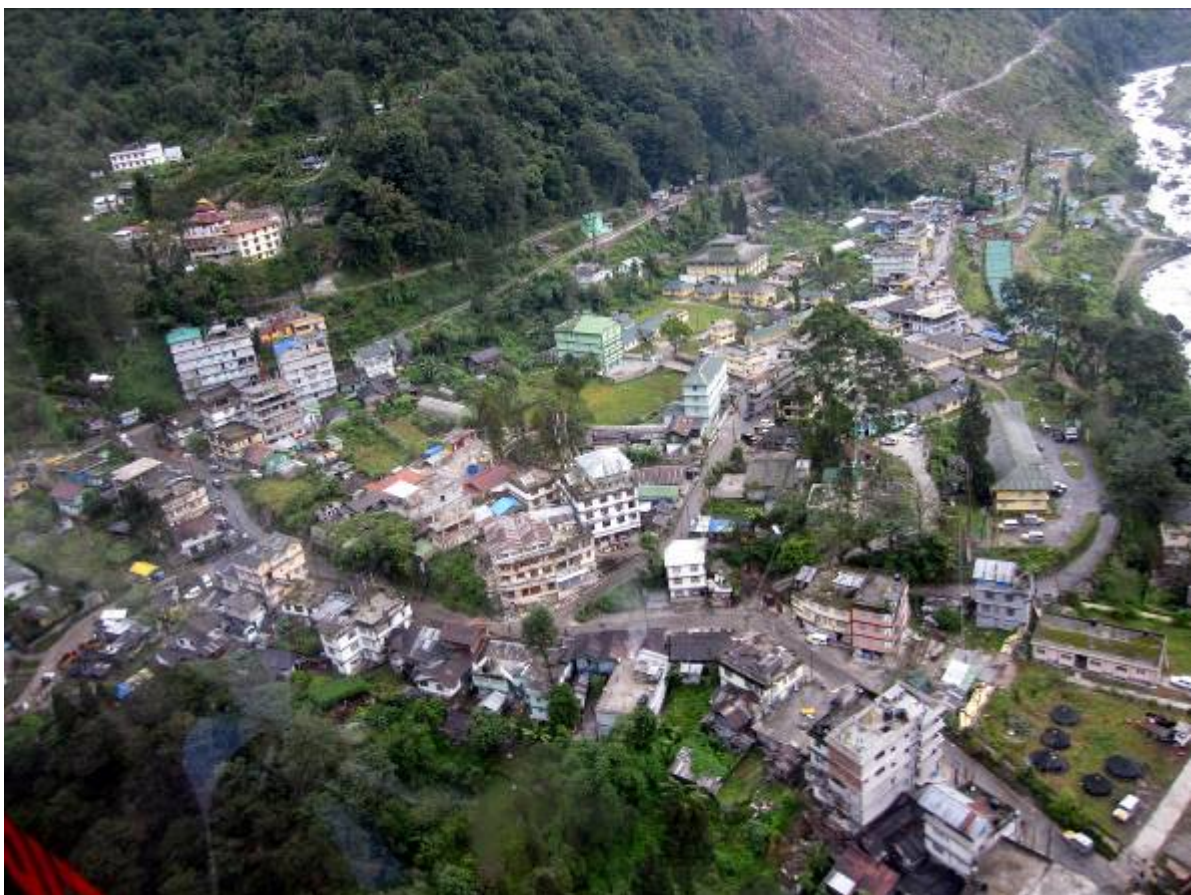
Fig. 3. Aerial photograph of Chungthang showing damages (Photo: Durgesh Rai)
