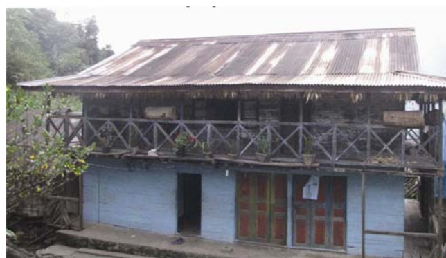
Figure 3. Traditional houses are typically two-storeyed, with framed structure made from woven bamboo or wood having a light CGI sheet roof.
