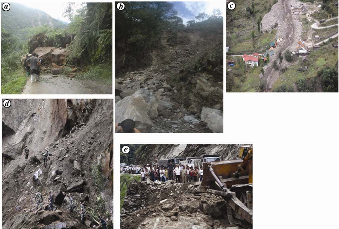
Figure 1. Weak geology, fragile ecology and heavy rainfall all combined to amplify the impact of the earthquake resulting in thousands of natural calamities in the form of landslides and slips, boulder falls and flash floods and causing colossal collateral damage. a , Boulder falls. b , Landslides. c , Flash flood in Lachung, North Sikkim. d , Cliff caves in on the national highway. e , Landslides block the national highway.
