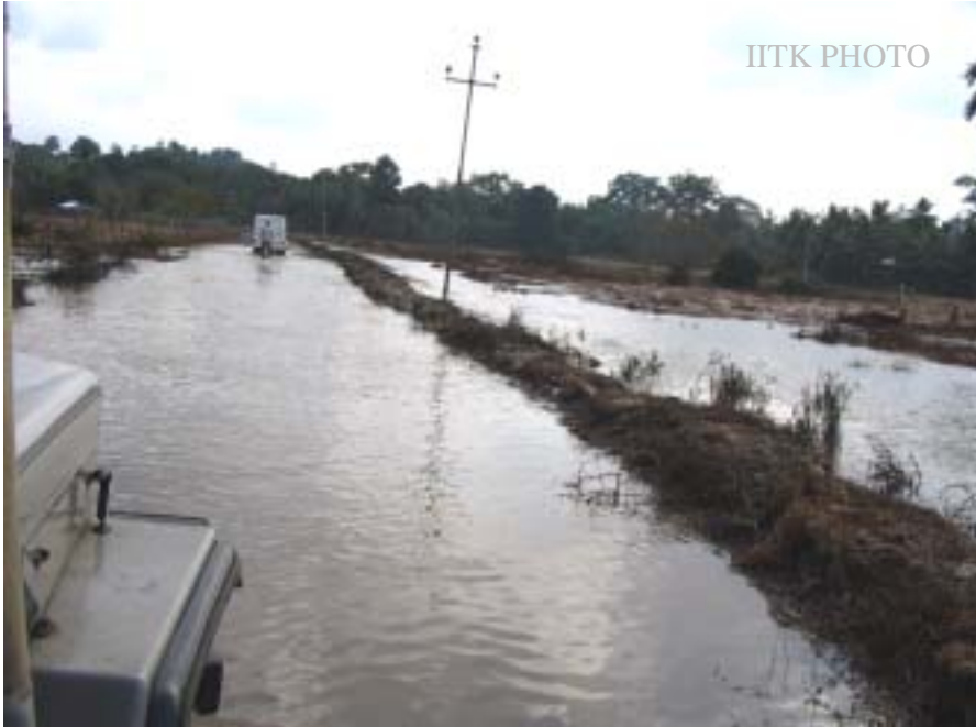
Figure 5: Sea water flooded ATR at Sipi Ghat area near Port Blair during high tide. (Photo: Goutam Mondal)
