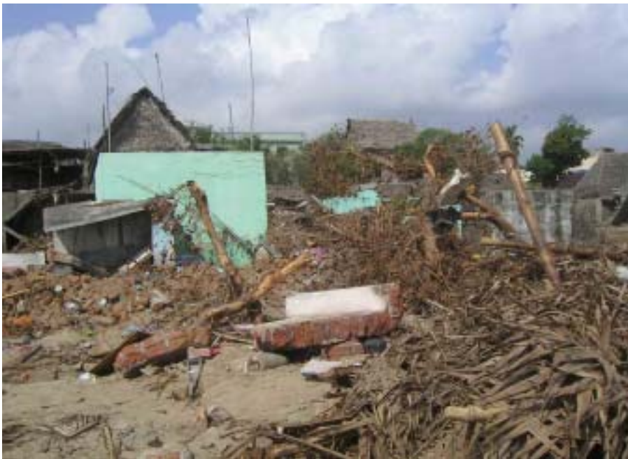
Figure 8: Ravaged houses at Nagapattinam due to poor constructions. (Photo: Alpa Sheth)
