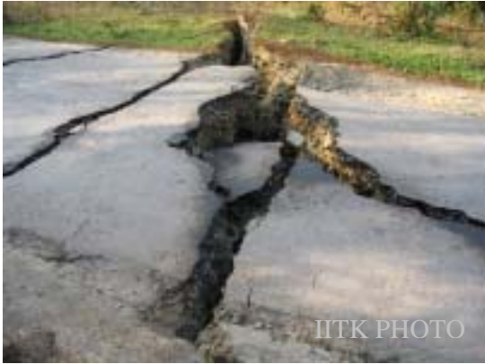
Figure 7: Ground deformation at Jarawa Creek, Baratang Island, Middle Andaman, (a) Damage to road connecting Baratang and Baludera Beach, (b) Splitting of a tree trunk due to ground rupture ( \approx 1.2 m wide). (Photo: Goutam Mondal)
