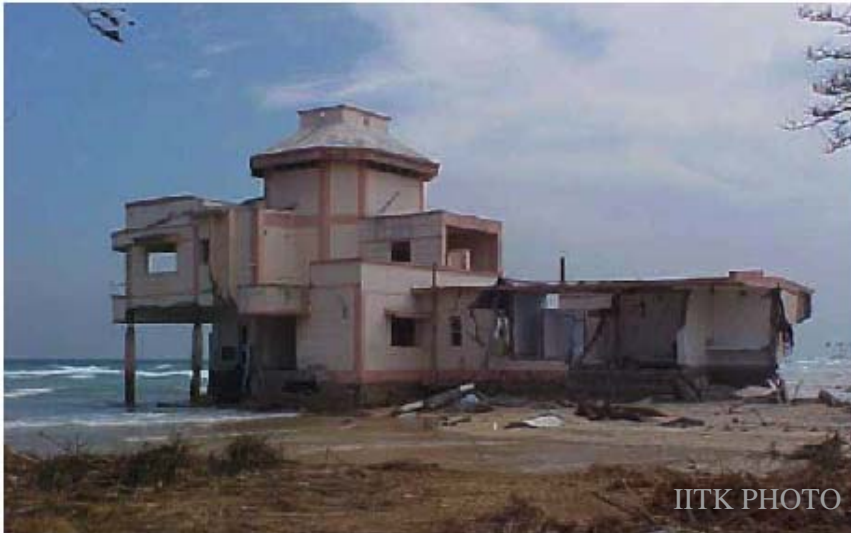
Figure 3: RC frame building (MES Inspection Bungalow) now stands in waters at the Military Residential Colony south of Malacca on the east coast of Car Nicobar Island. (Photo: CVR Murty)
