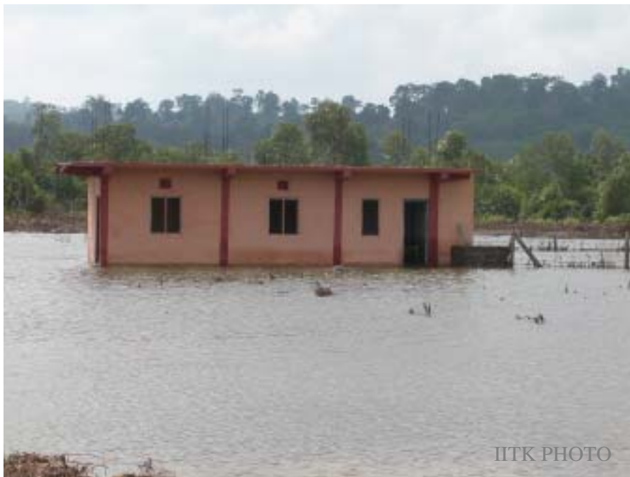
Figure 4: Sea water level at Port Blair with respect to land has gone up by about 1.0m. Hence, many areas are now flooded during high tide (Photo: Sudhir K Jain)
