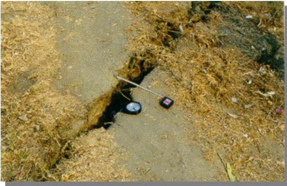
Figure 5: Ground fissure at Telecom Hill near Gopeshwar
