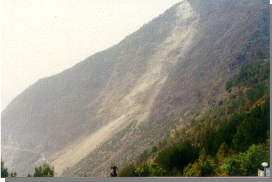
Figure 6: A major landslide about 1km north of Gopeshwar. It blocked the road traffic to Okhimath for a considerable period.
