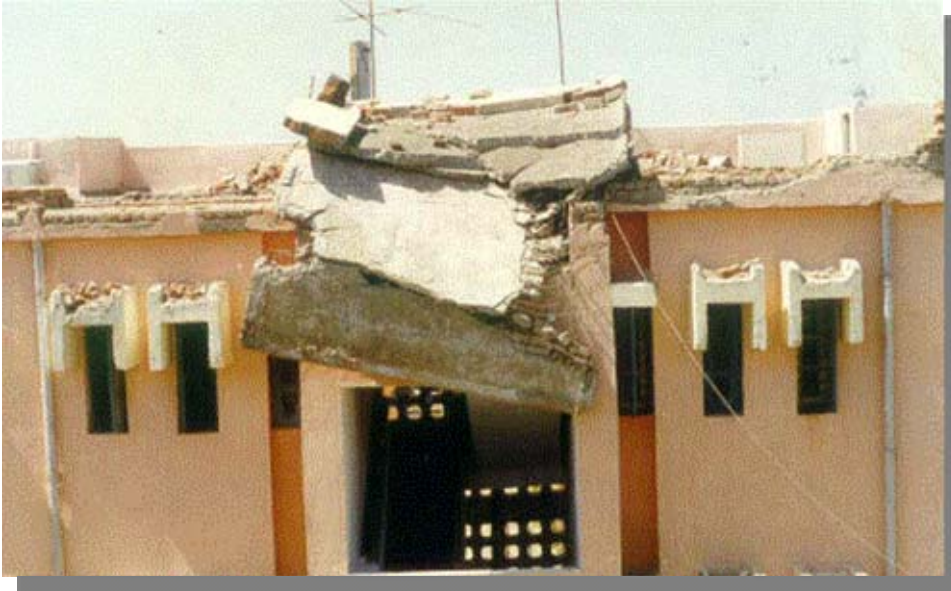
Figure 5 - Many staircase towers, called "mumty," which project about 2 m above the surrounding construction in masonry houses, collapsed.
