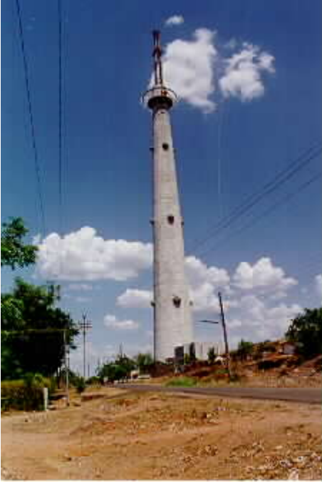
Figure 8 - No damage was observed to the 225 m high RC and steel TV tower in Katanga.
