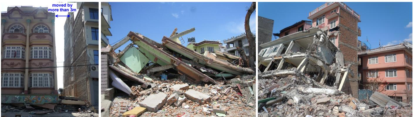
**Fig. 1.** Collapse of multi-storey buildings in Kathmandu
