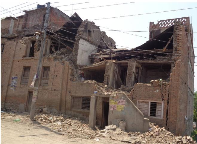
**Fig. 2.** Collapsed unreinforced masonry buildings at Bhaktapur
