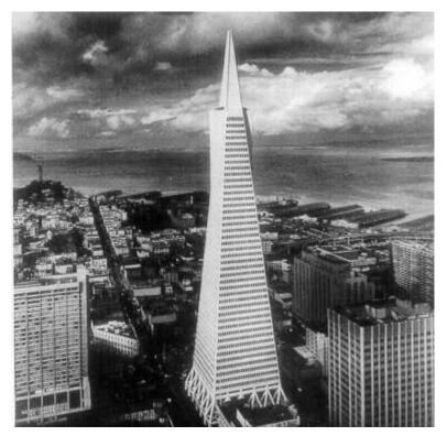
Though the top floor of the 49-story Transamreica Pyramid swayed more than one foot from side to side in the 1989 San Francisco earthquake, no one was injured nor the building damaged. Casualties were comparatively few in that quake. Most houses that collapsed were built on unstable ground.
